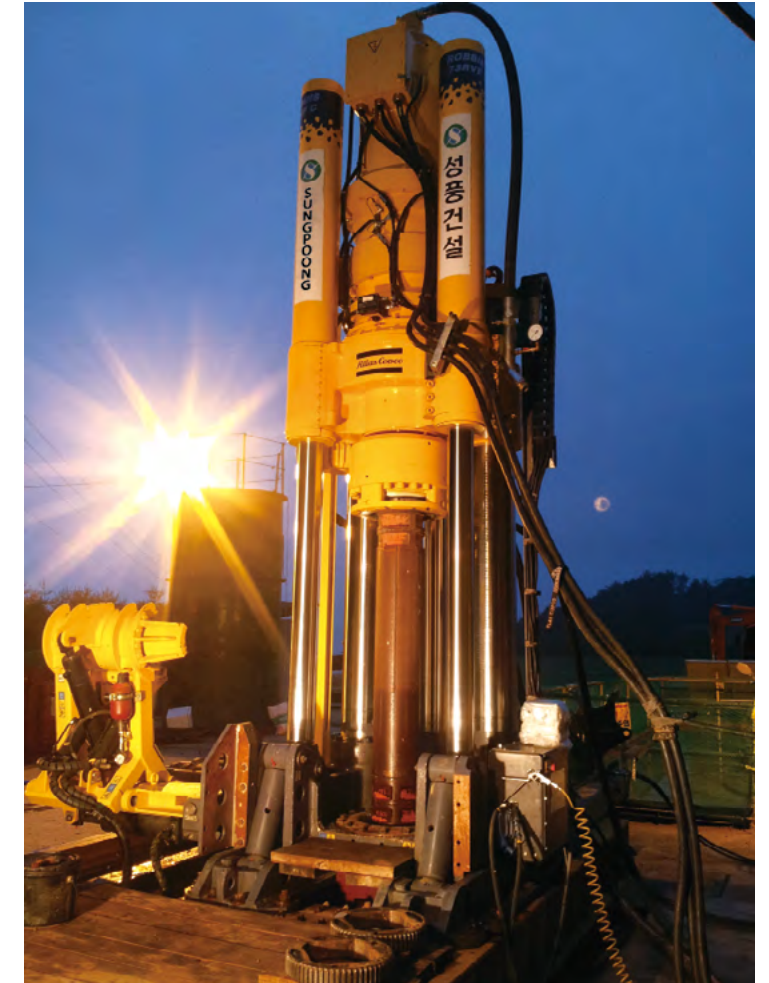
Pilot Hole Excavation
