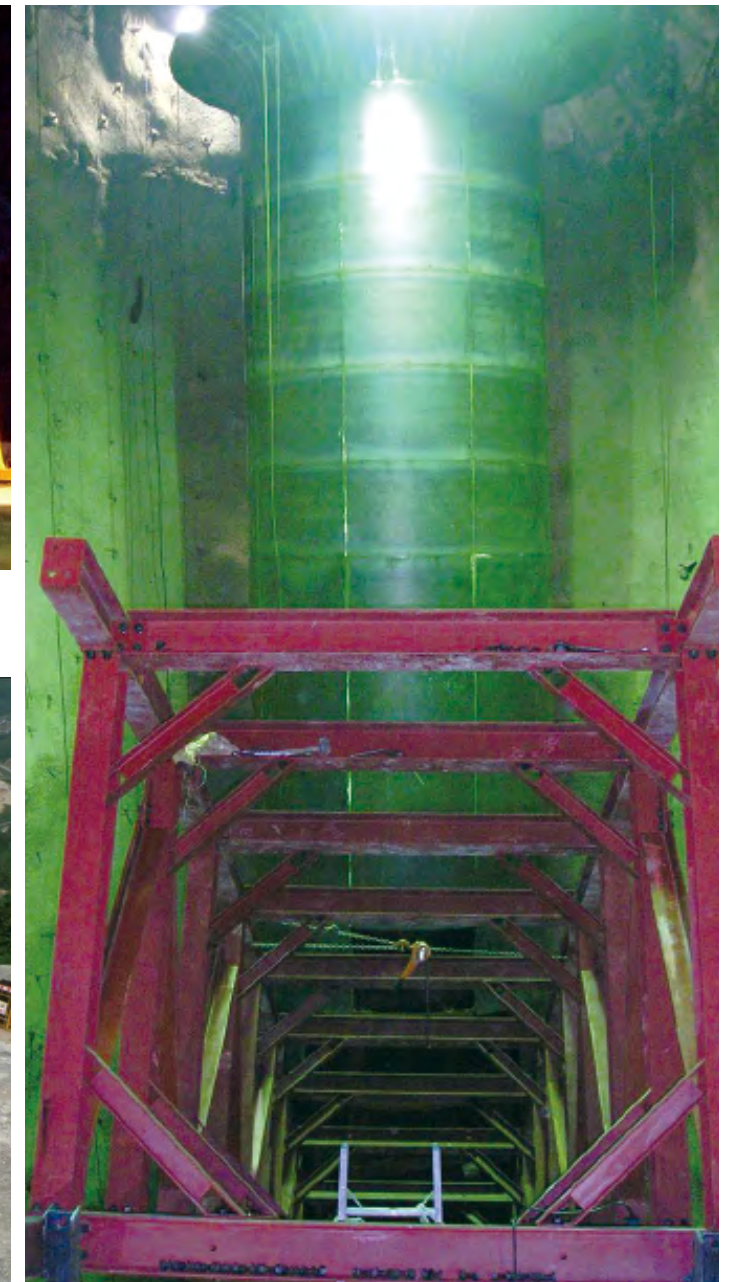
Orifice at Cheongsong Pumped Storage Power Plant
