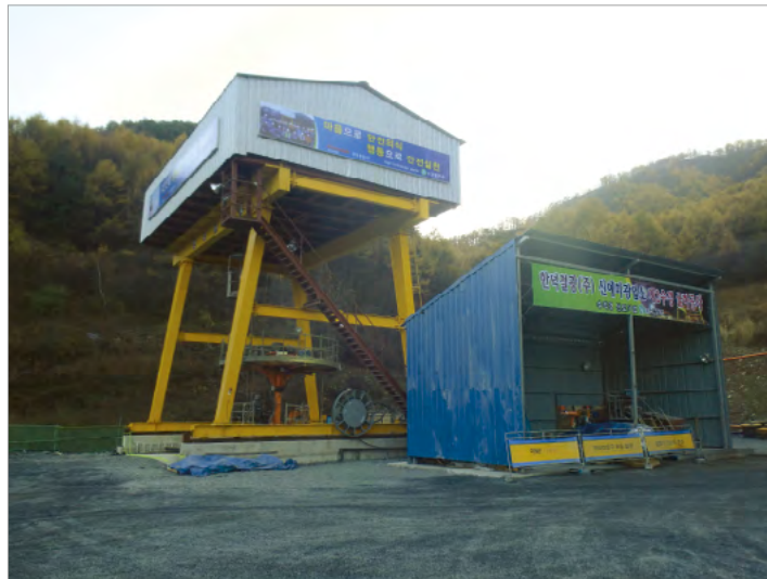
Upper Gantry Crane (Handuk Iron Mine)
