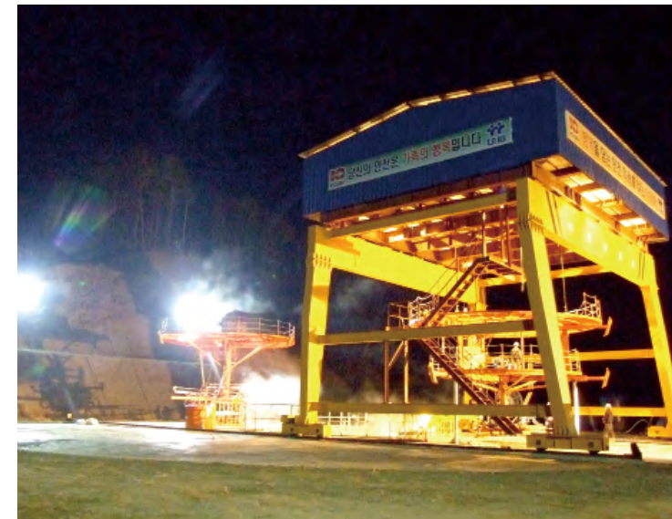
Gantry Crane at Yecheon Pumped Storage Power Plant Construction Site
