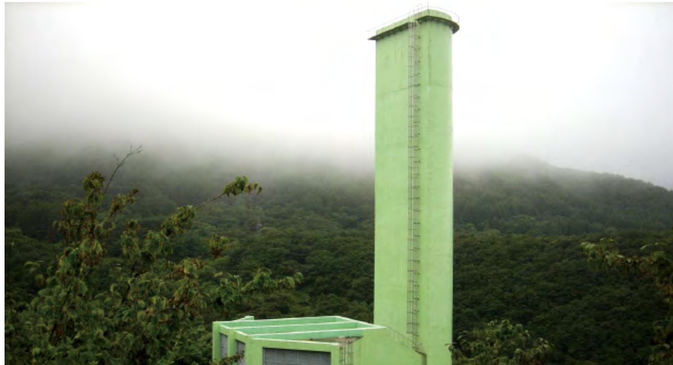
Ventilating Shaft at Jukryeong Tunnel
