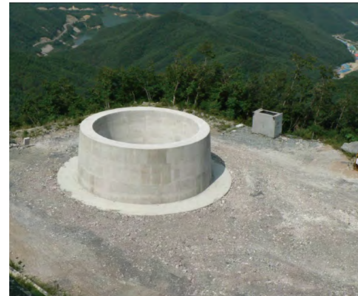
Surge Tank Structure at at Cheongsong Pumped Storage Power Plant
