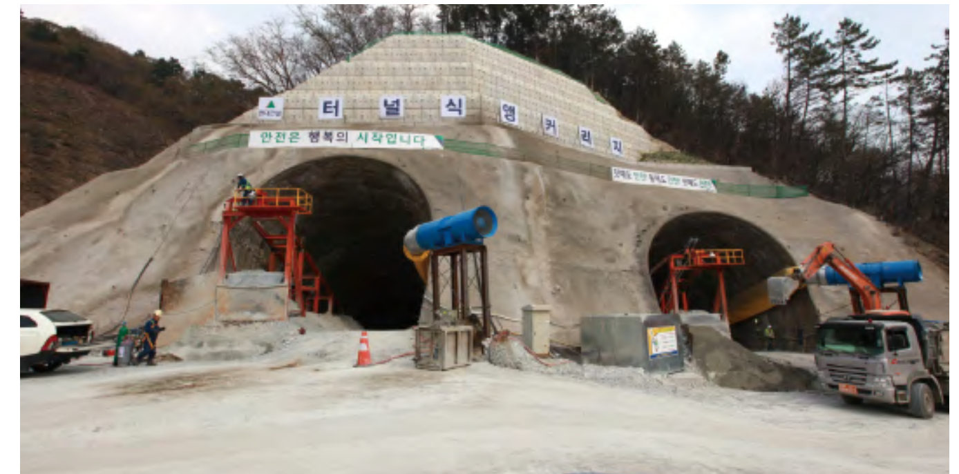
Tunnel-Type Anchorage Construction Site Whole View(Ulsan Bridge)
