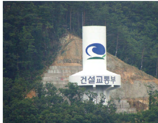
Ventilating Shaft at Nungdong Tunnel
