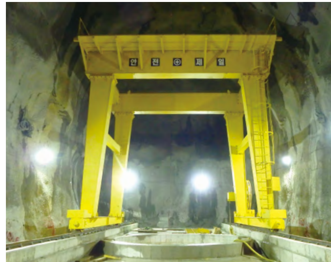
Lower Gantry Crane (Handuk Iron Mine)
