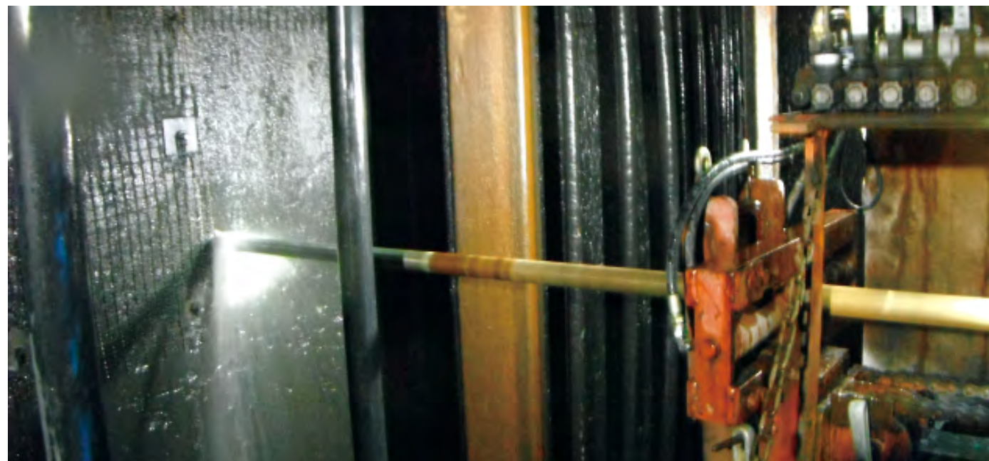
Vertical Shaft Sidewall Reinforcement work (Jangseong Mining Office of Korea Coal Corporation)
