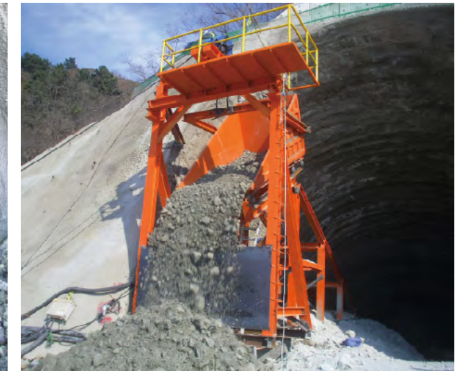
Muck Disposal by Skip Equipment
